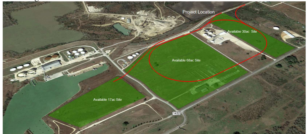
The new rail from the Rail Expansion Project is marked in red and available lease site is highlighted in green.
